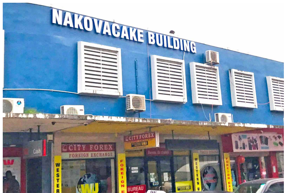
Nakovacake Building in Nadi Town
