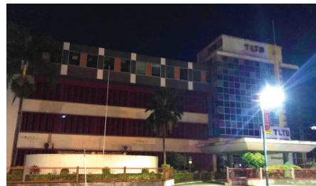
Image of the TLTB Building which reveals that lights were switched off during the Global Earth Hour event on the 24th of March 2018
