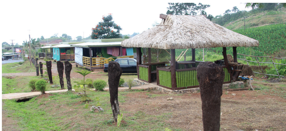
The first three housing built by Climate Forest Investment in Tacirua which was initiated by the Mataqali Naulukarua in Kalabu, Naitasiri with the support of TLTB
