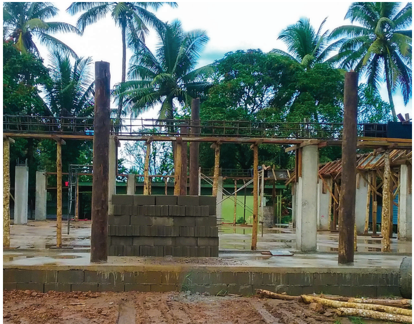
Hall construction progressing well at Vunivivi
