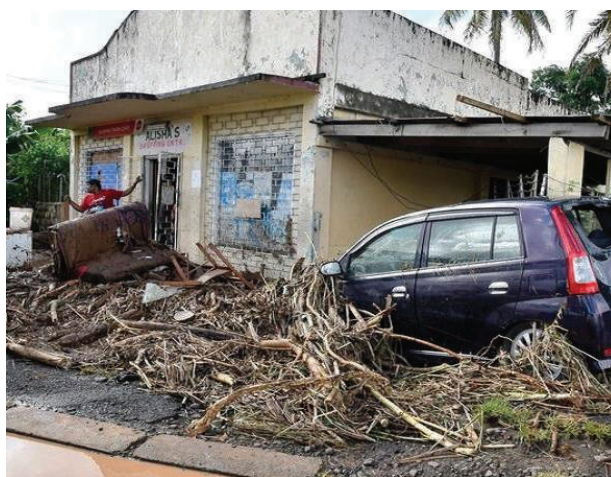
Commercial and agricultural properties were damaged during Hurricane Josie and Gita
