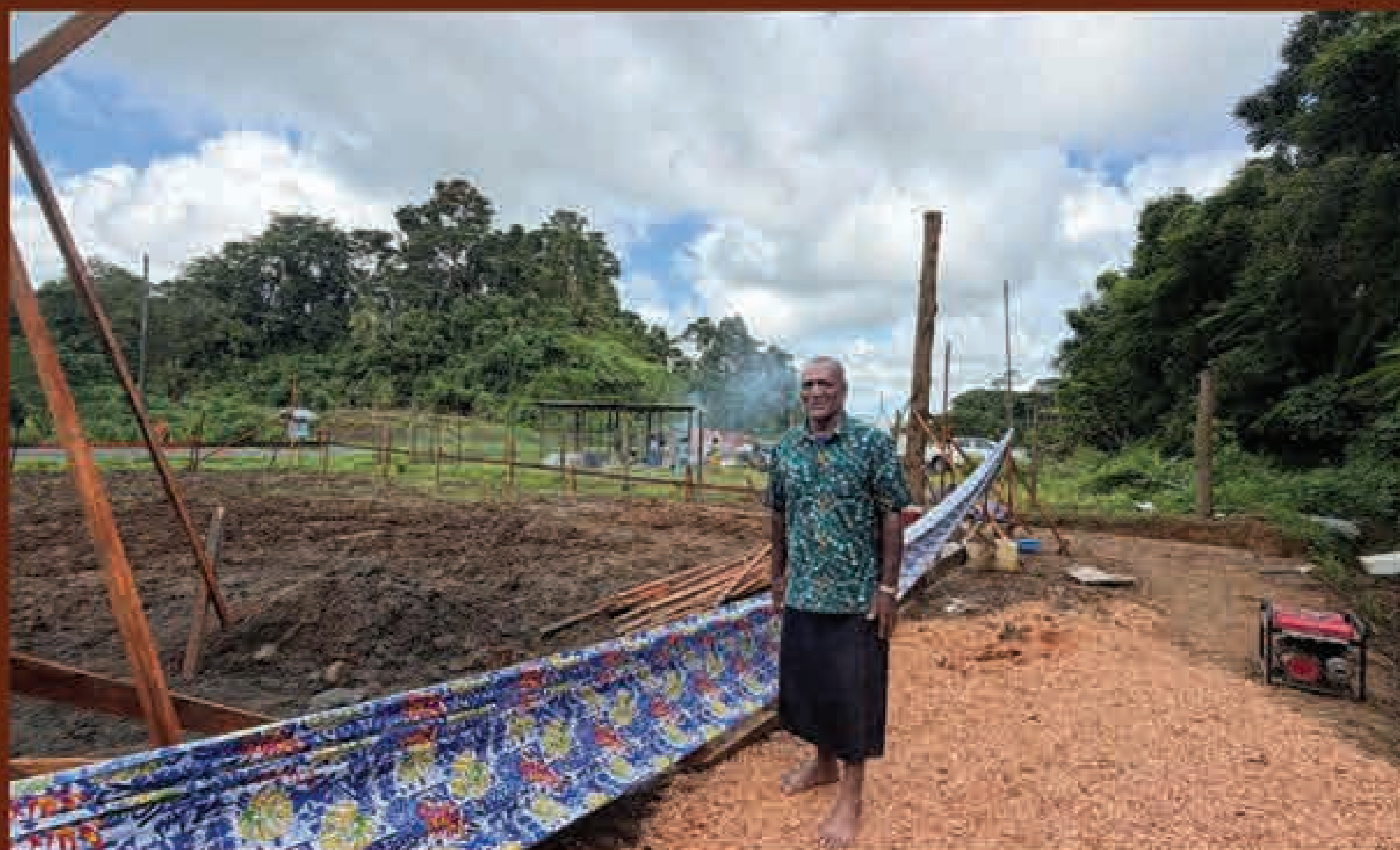
Kobakobau Investment securing an industrial lease at Kasavu
