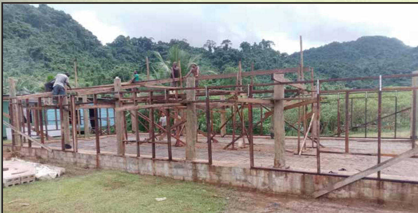
Community hall construction by Mataqali Waisali
